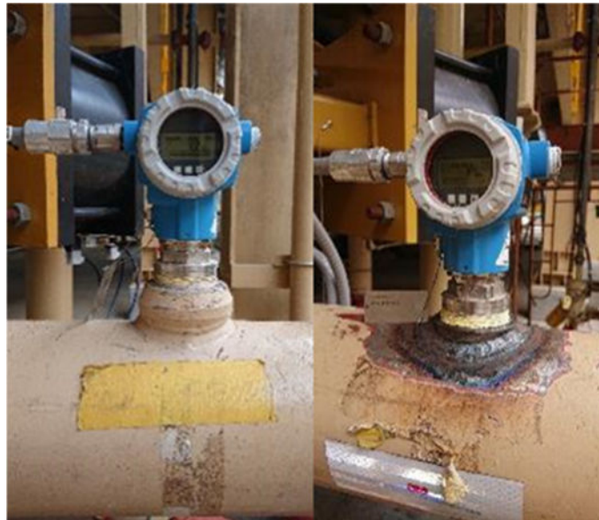
Figure 14 Flush mounting instrumentation to eliminate cemented blockages
